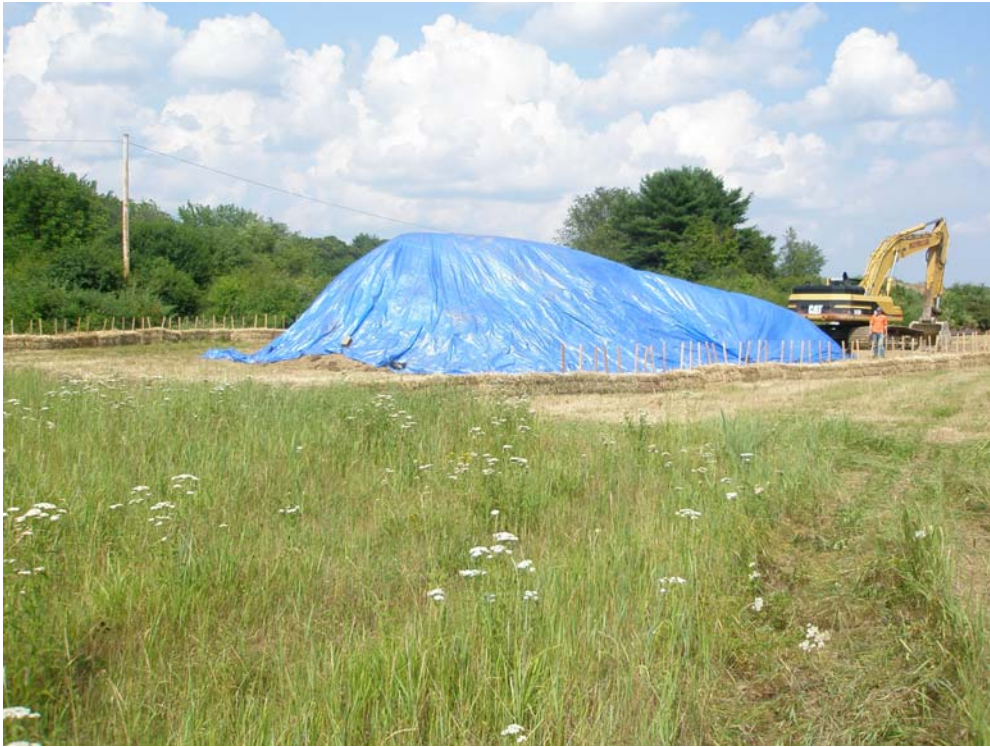
Photograph 3 – Clean Soil Staging Area
