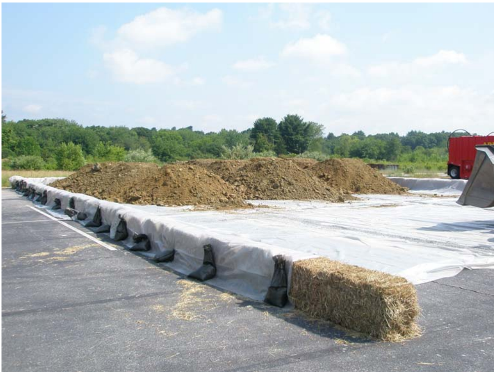
Photograph 2 – Lined Stockpile Area in Parking Lot
