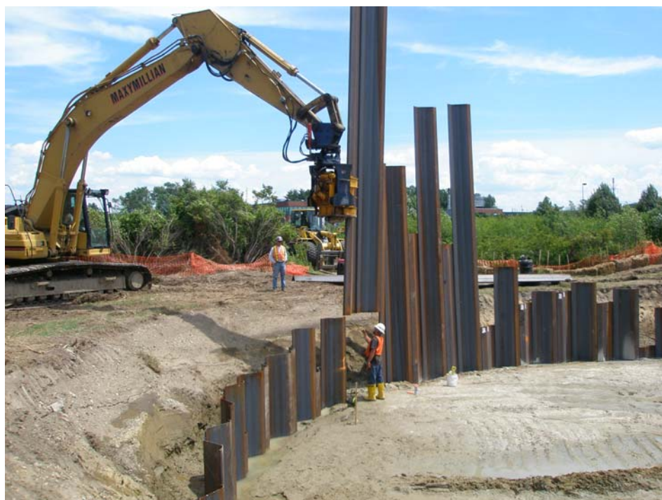
Photograph 6 – Installation of Last Sheetpile
