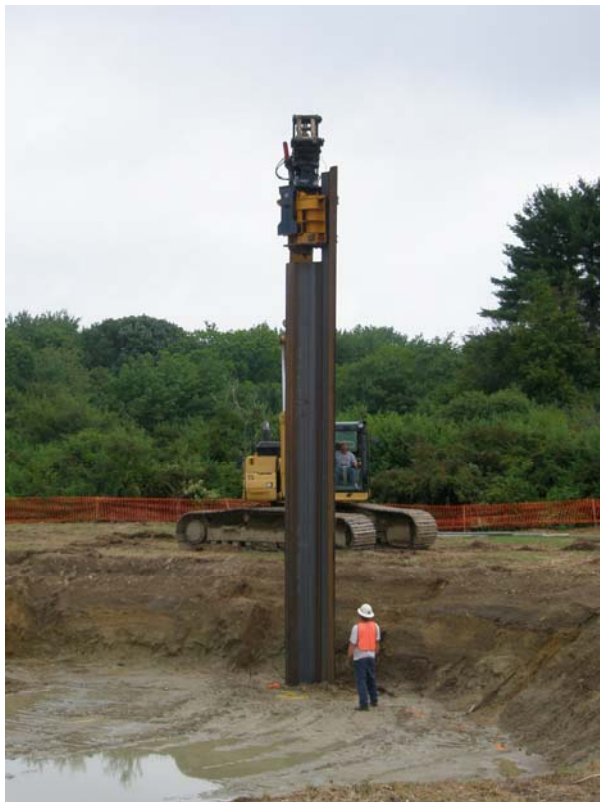
Photograph 5 – Commencing Pile Driving
