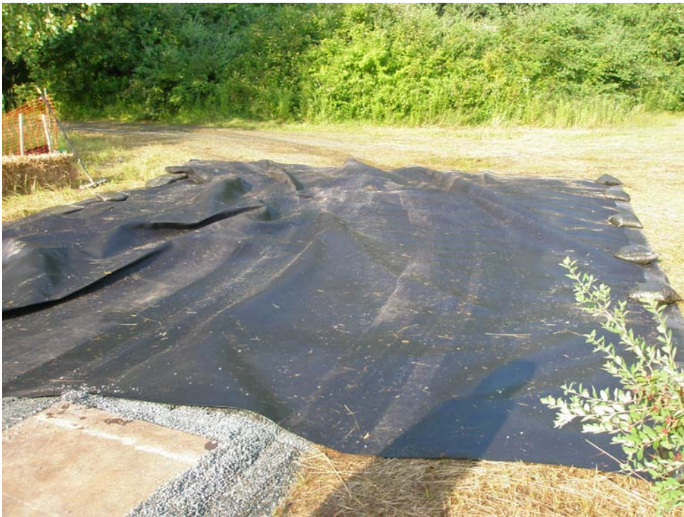
Photograph 4 –Decontamination Pad on Cart Path
