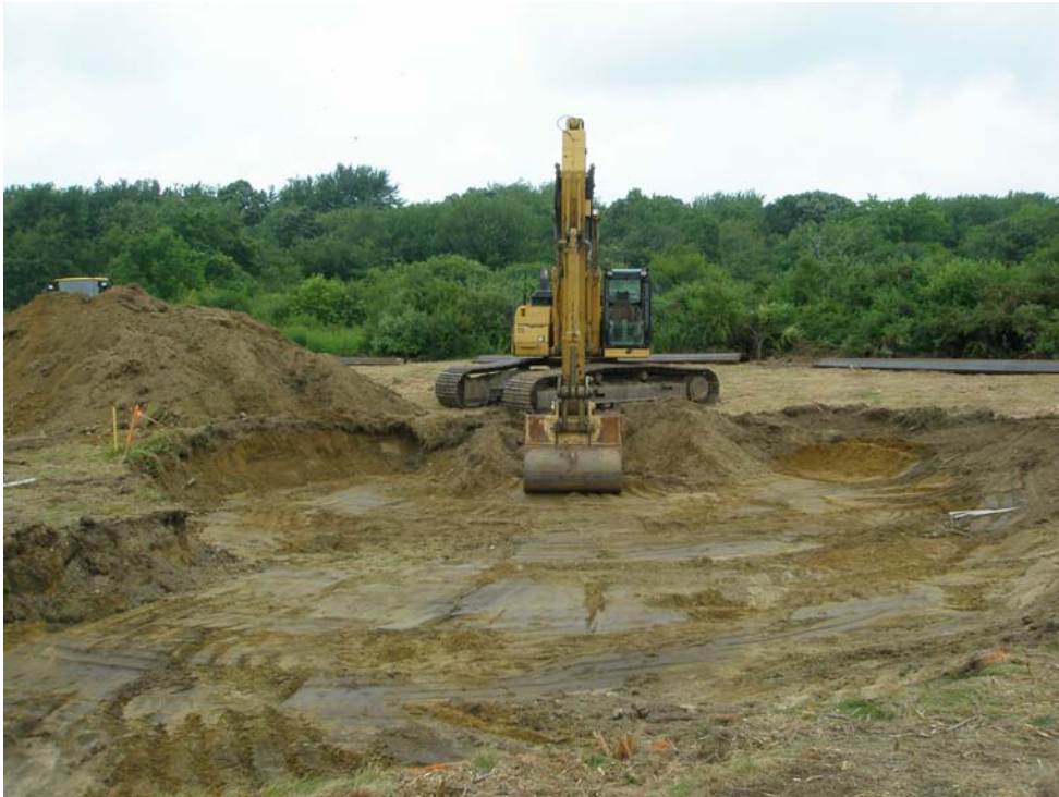
Photograph 1 – Excavation of Cofferdam Area
